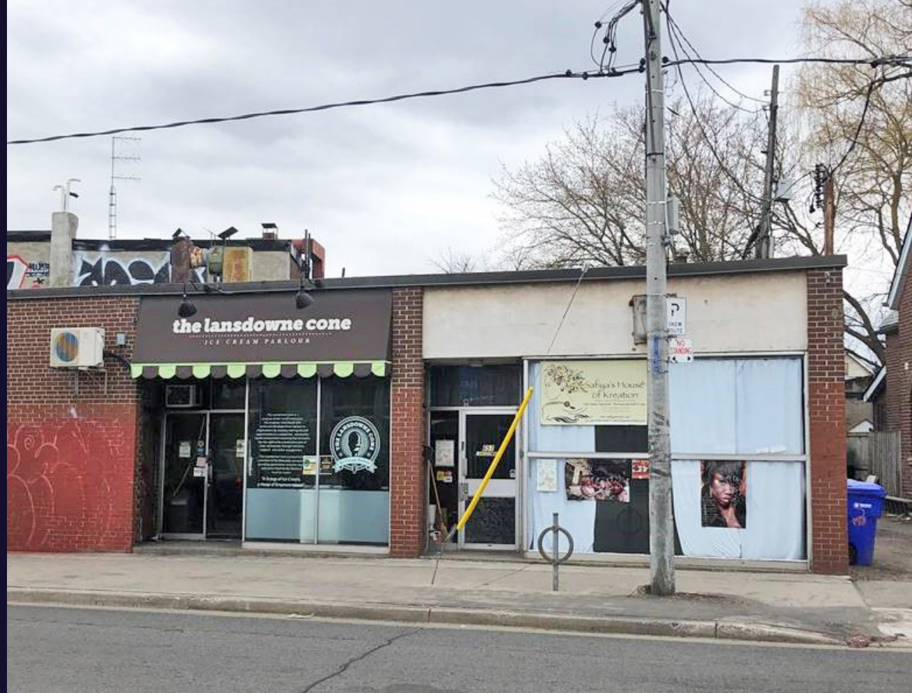
1287 BLOOR STREET WEST UNITS 2&3
