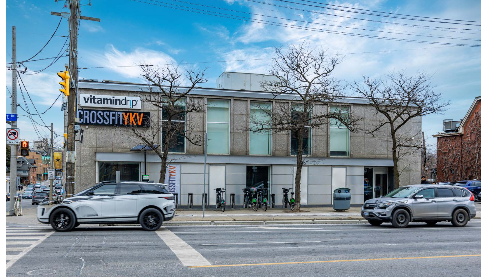
DAVENPORT ROAD FRONTAGE
