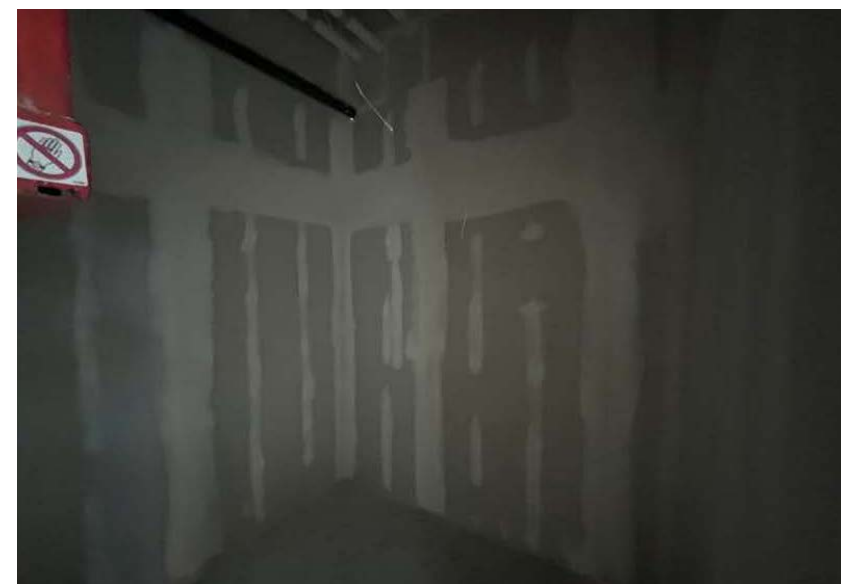
Electrical room taping
