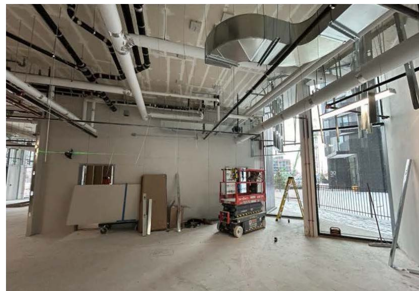
Framing and boarding of consult 141 and screening 140
